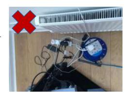
It is recommended to use a multi-way extension lead instead of a block adaptor. Some block
