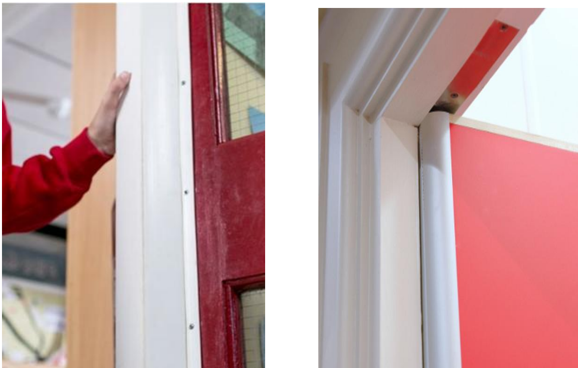
Pinch points removed from existing doors by installing hinge guards or installing new doors with integrated hinge guards.
