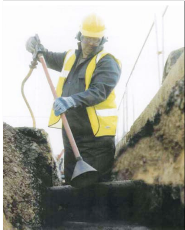
Figure 7 Using an air digging tool
